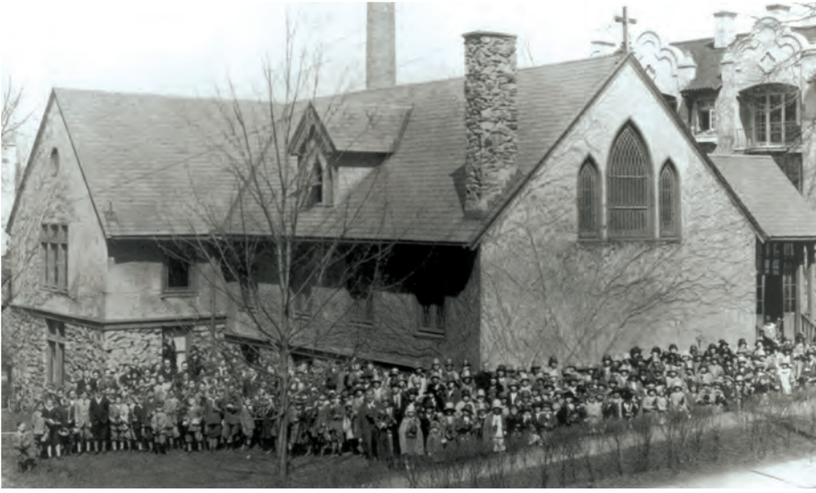
WOODEN PARISH HOUSE, 1924. Sunday school children gather in front of the parish house just before it was taken down to make room for the new church.
